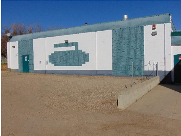
New curling club built by the Town of Legal 1977
